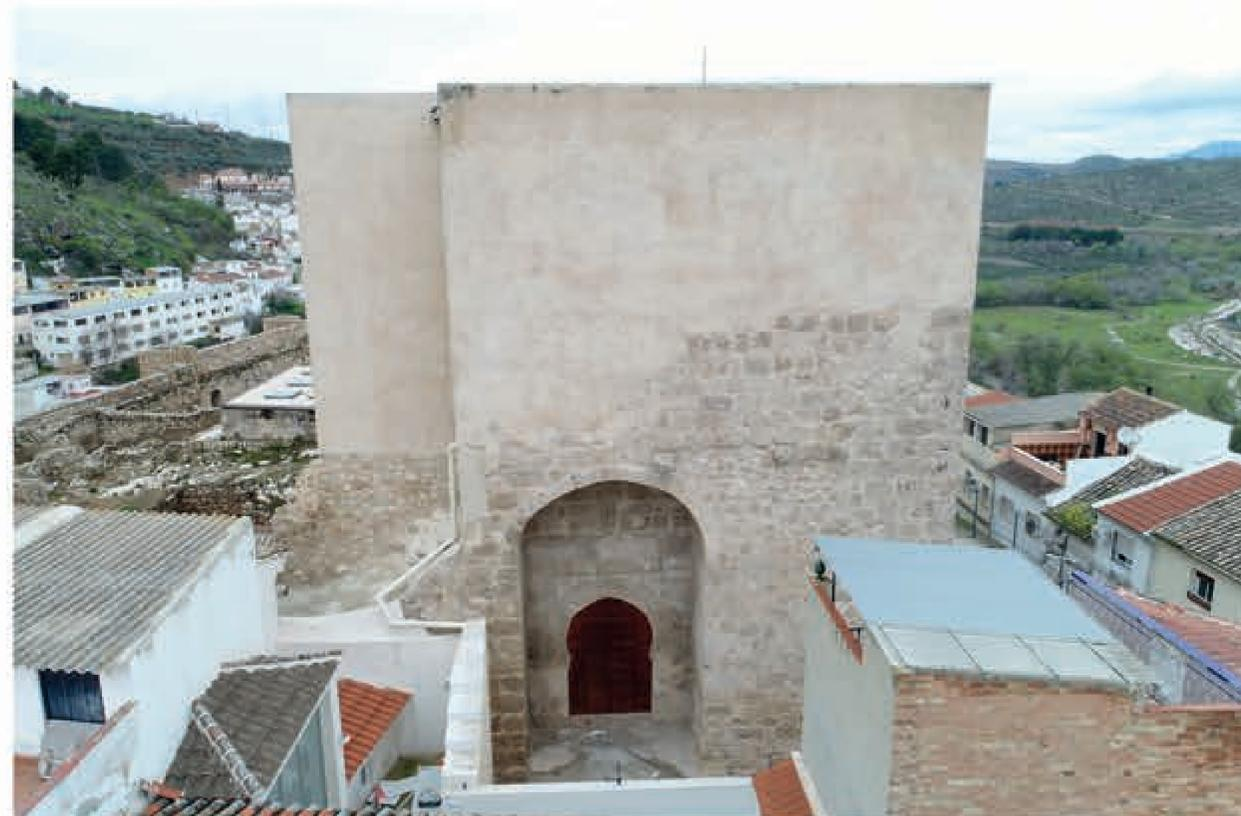
To the west of this tower and accessible through an opening in its wall, is the building known as *Caserón de los Alcaldes*, built by Pedro de Tapia in 1616. It has a trapezoidal shape, with the average dimensions of 23.80x7.30 m, and is built with masonry walls, using brick in the openings of doors and windows.
